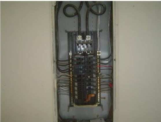
Main electrical disconnect breaker is located in panel box in garage. Cover does NOT have to be removed to access disconnect.
