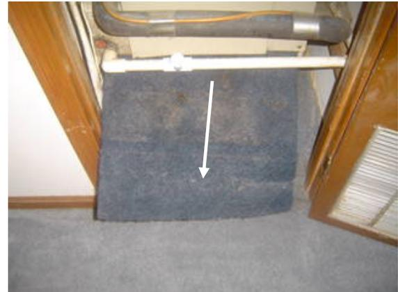
The a/c filter is located in the bottom section of the air-handler. Filter should be changed periodically (30-90 days) as required.
