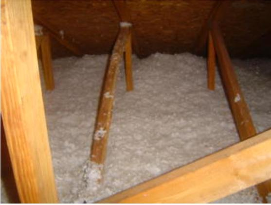
Blown insulation in the attic areas appears to provide an approx. insulation value of R-19 (minimum required when house was built).
