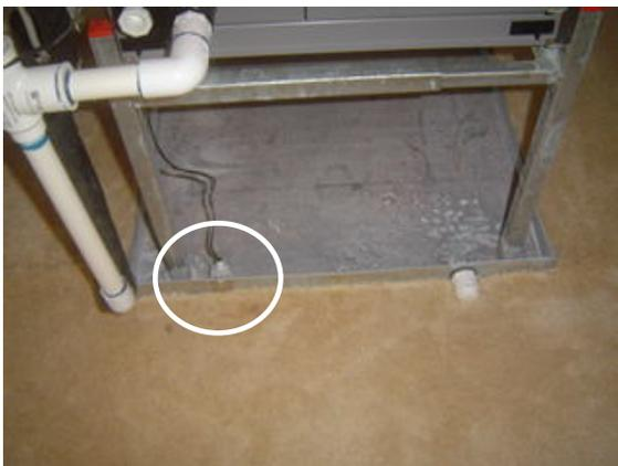
Close look at example of catch-pan and high-level shutoff switch combination used to control condensate overflow
