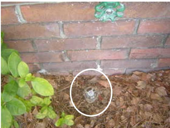
Close look at water shutoff valve on the front of the house to the left of the garage door. Water can also be shutoff at the meter if required.
