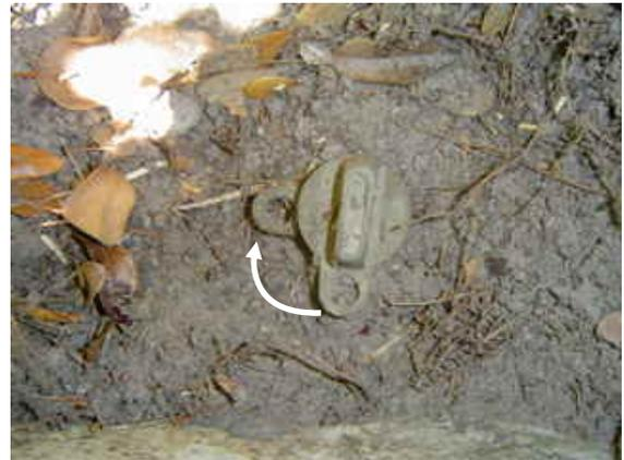
Shutoff of water at the meter is done using a wrench by turning the brass valve on the city side of the meter so that the rings line up.
