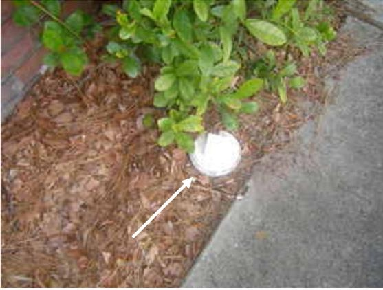
Main sewer cleanout is located in the front planter bed. Cleanout is important to the homeowner if the drain lines (toilets, sinks, etc.) become clogged. Uncap cleanout. If standing water is noted in the pipe the clog is probably between the cleanout and the street. If there is just a trickle or very little water in pipe the clog is probably between the fixture (toilet, sink, etc.) and the cleanout.
