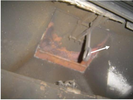
Close look at chimney flue damper control on the damper located at the chimney throat inside the fireplace; pull handle to open damper. The flue damper must be open whenever the fireplace is in use.
