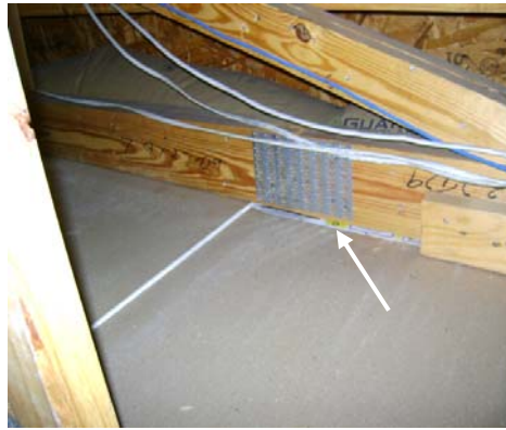
Paper edge tape label on the ceiling drywall is found along bottom truss cords in the attic.
