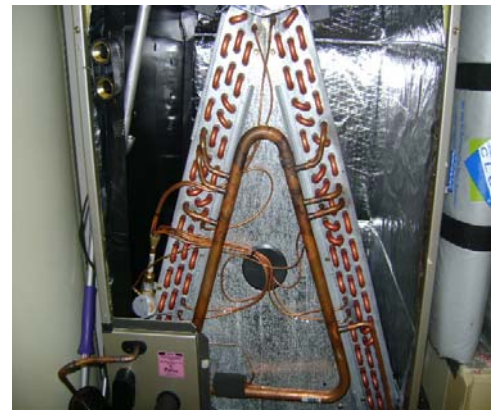
The discolored and “black” copper air-handler coil components in the left-hand picture have been exposed to the corrosive effects of the various gases given off by the Chinese drywall; compare bright copper air-handler coil components in the right-hand picture.
