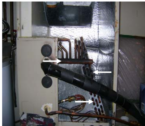
The discolored and “black” copper air-handler coil components in the left-hand picture have been exposed to the corrosive effects of the various gases given off by the Chinese drywall; compare bright copper air-handler coil components in the right-hand picture.
